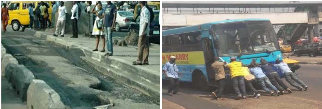
(a) Bad road section (dedicated BRT lane) 2 (b) BRT bus being pushed by its passengers
